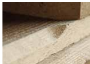
Haunches on bottom planks
